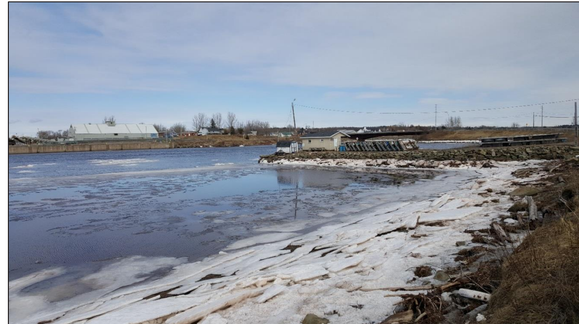
Photo 1. The proposed Project area looking east.
